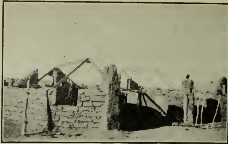
FIG. 6.—Frames for tents on adobe walls.
